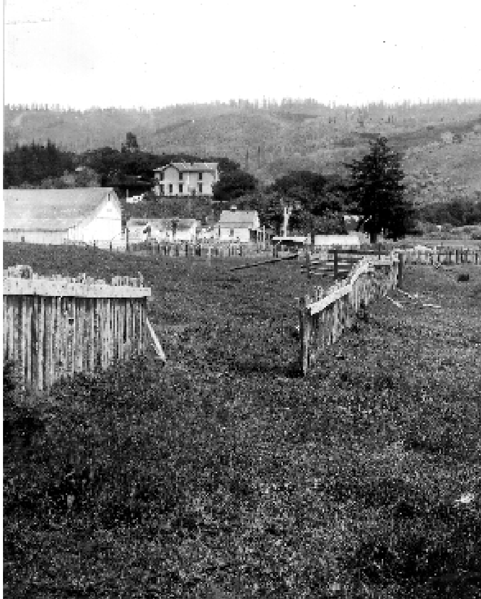
1906 earthquake rupture with large ground displacement. Notice that the farm buildings were largely intact.
